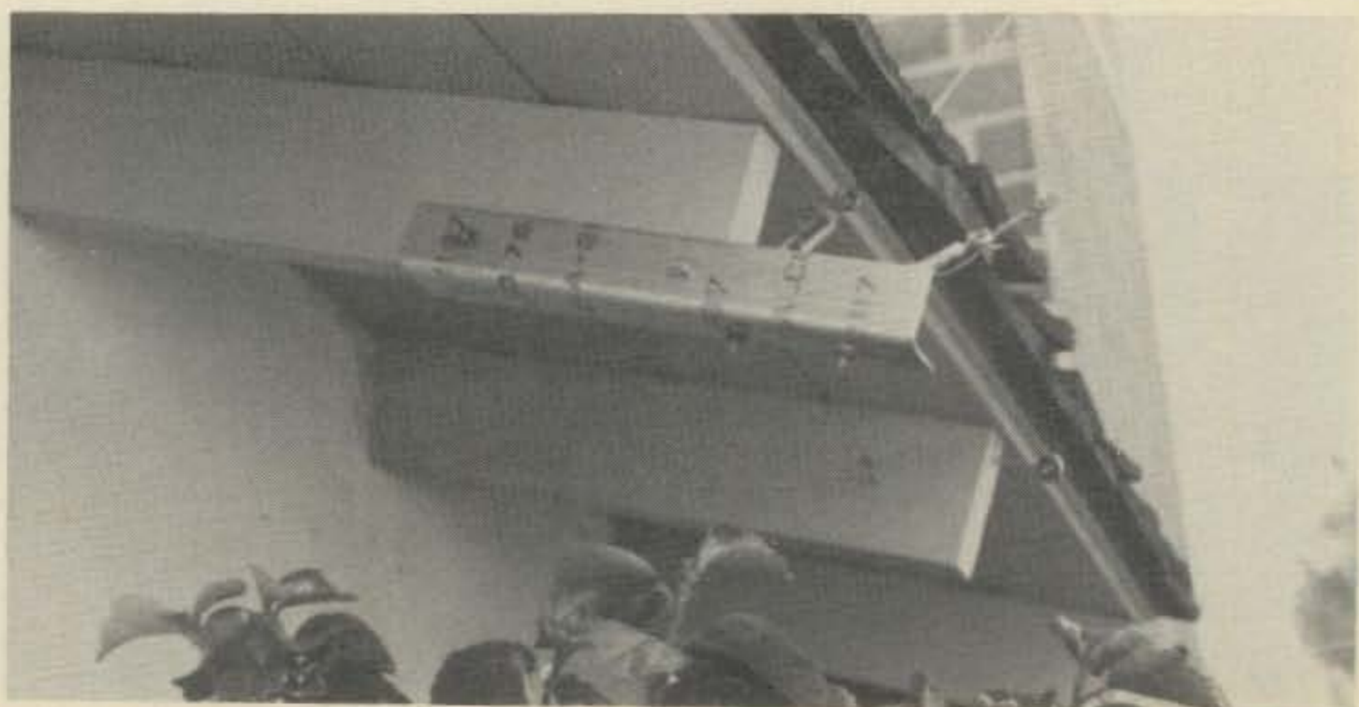
This photo shows how the guy wires are mounted under the eave of the house.
